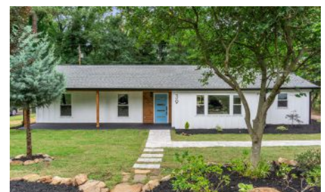
Entire House $500,000 to $750,000 Liv Companies, LLC A NARI Accredited Remodeling Company® Burr Ridge, Illinois
