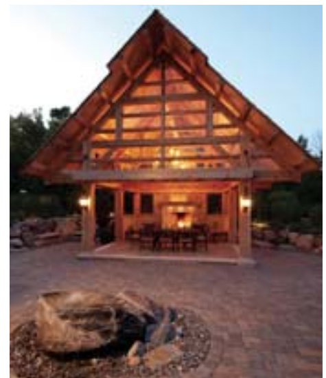
TOP: A spacious terrace, ringed by large boulders, extends the outdoor living area beyond the more protected refuge the gazebo offers. ABOVE: Gable-end windows bring lots of light into the sheltered structure while keeping the gazebo more insulated than a totally open design would allow.
